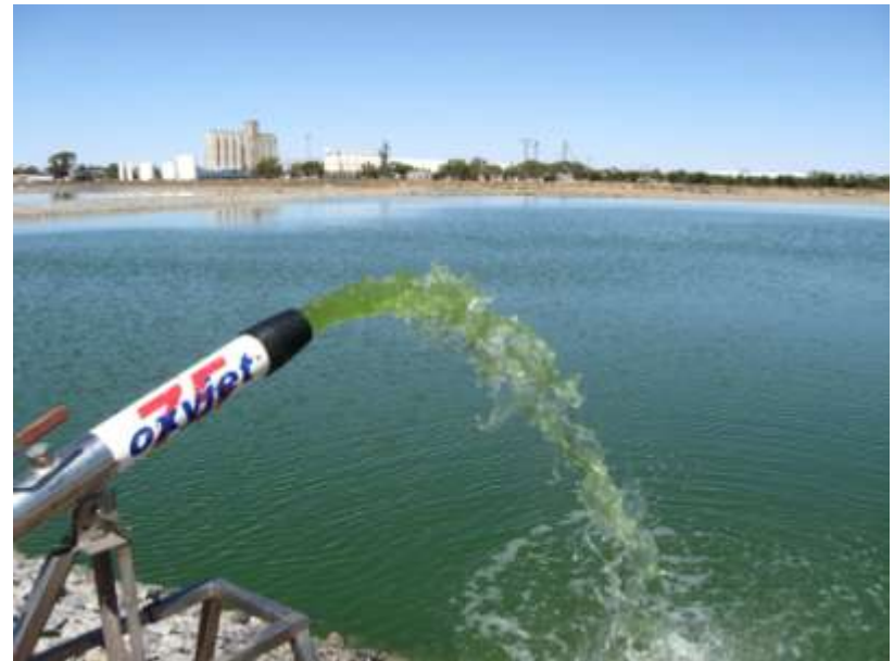
Merredin WWTP (Barrington 2009)
